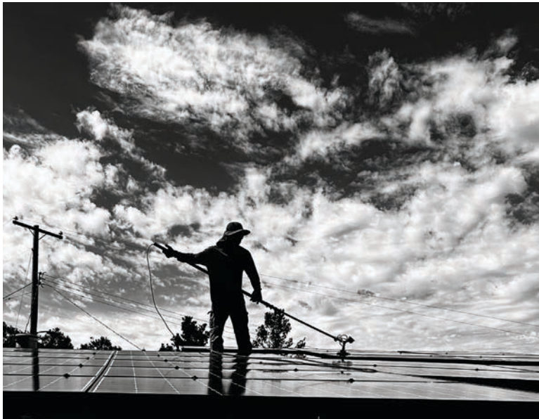
Cleaning Solar Panels
