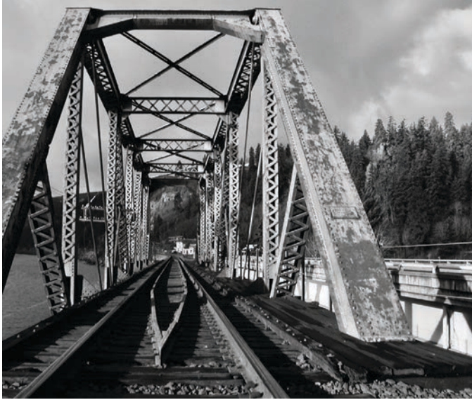
Railway Bridge, Lake Oswego, OR
